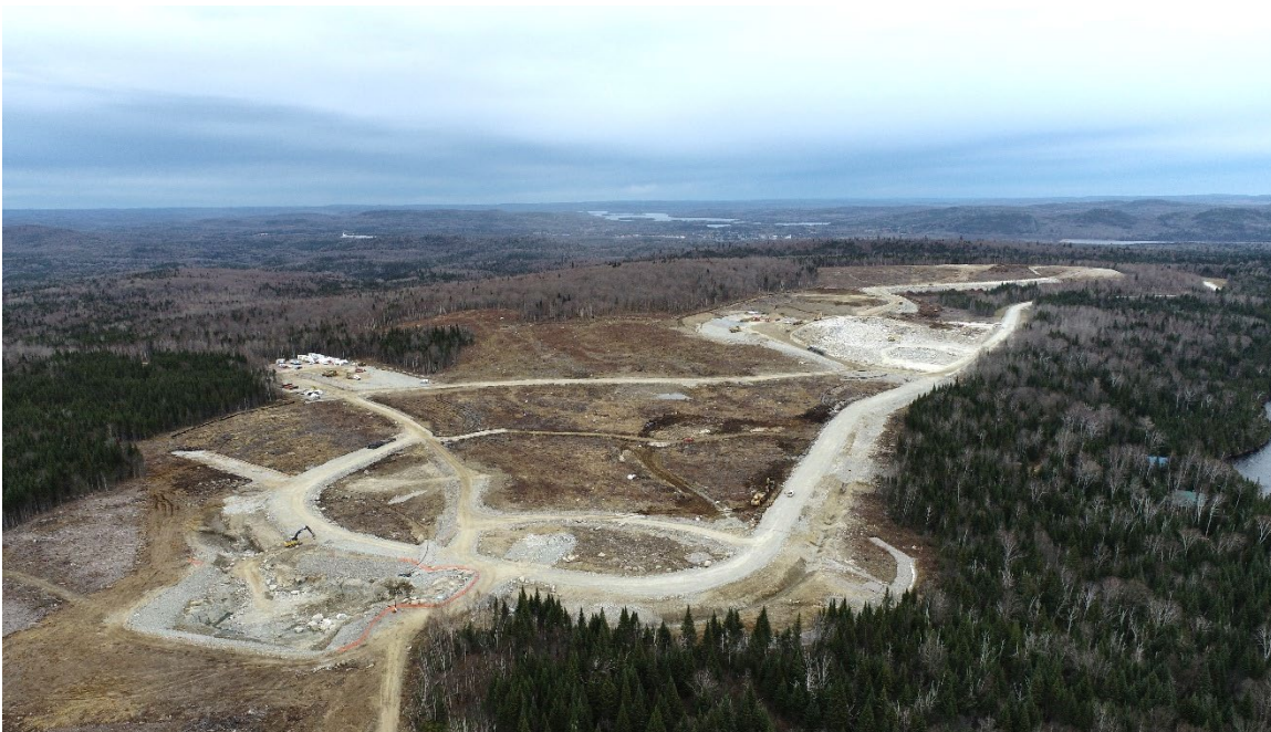
Aerial view of NMG's Phase-2 Matawinie Mine under construction.
