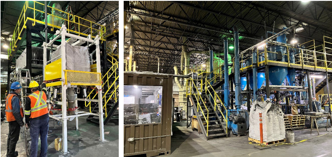
(LEFT) Workers review commissioning plans for NMG’s new Phase-1 shaping module.
