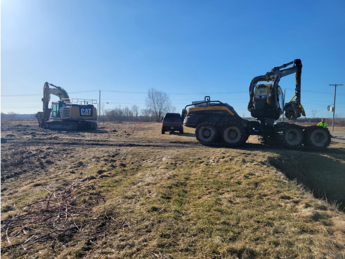
Tree clearing operations at NMG's Phase-2 Bécancour Battery Material Plant site.
