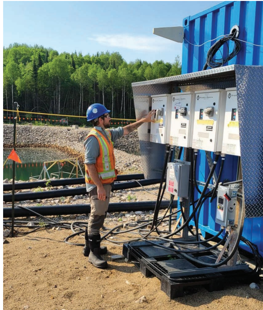
David, Environment Technician at the Matawinie Mine, starts pumping operations at our Phase-1 water treatment plant.
