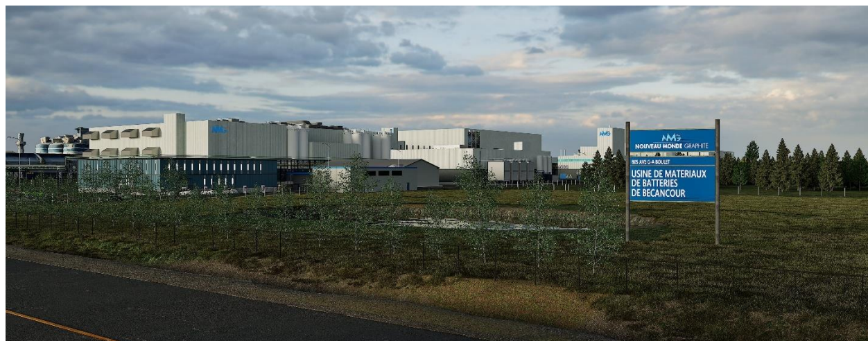
Figure 1 – Computer-Generated Illustration of the Planned Bécancour Battery Material Plant Project based on the 2025 Updated Feasibility Study
